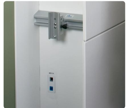
Side panels accommodate a variety of configurable services. Smooth face panels are lap jointed to help prevent liquids from seeping behind panels.
